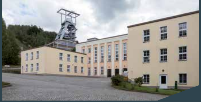
Shaft Complex 371 near Bad Schlema (element 38)
