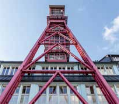
Arno-Lippmann-Schacht (shaft), Altenberg (element 1)
